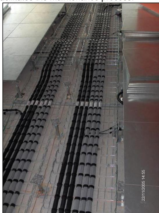
Figure 12. The use of cable tray under the raised floor (Frank Yang, Data Center Business Unit CommScope, Inc, 2010)
