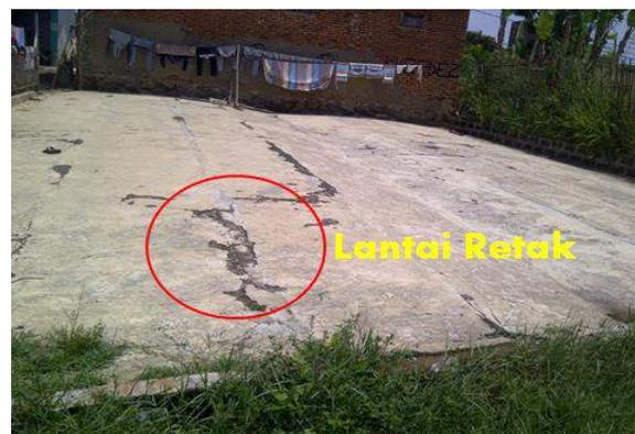
Figure 5. The Drying Floor before Construction
